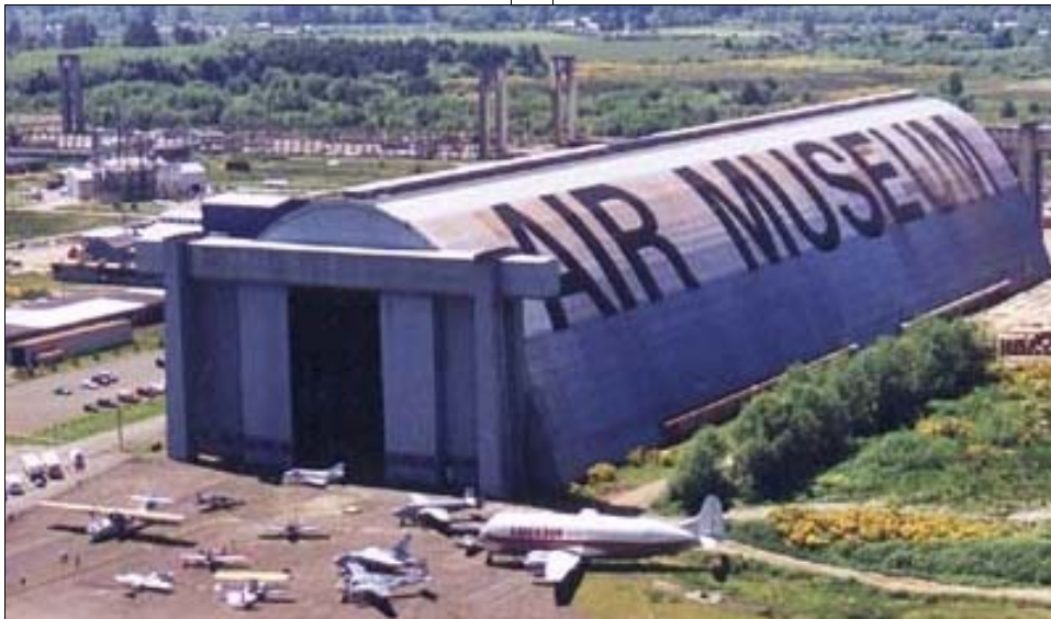
Blimp hangar that Felix, Maurice, and several of Felix's brothers worked on in 1942 is today an air museum. The hangar pictured above is one of two built near Tillamook to house a squadron of blimps used for coastal submarine patrol and convoy escort. The wood-built hangar is 1,072 feet long, 206 feet wide, and 192 feet high, with an indoor area of seven acres. Felix saw this hangar completed, then returned home to fetch his family. While he was gone a second was rushed to completion in 30 days. The second burned in down 1992. Photo used with permission of Tillamook Air Museum.
